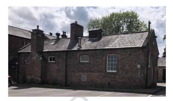
Hard cement mortar, with open and eroded joints and bricks Efflorescence on chimney breast Rainwater goods in very poor condition
